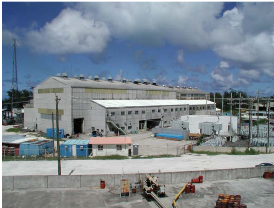
CUC Power Plant I
