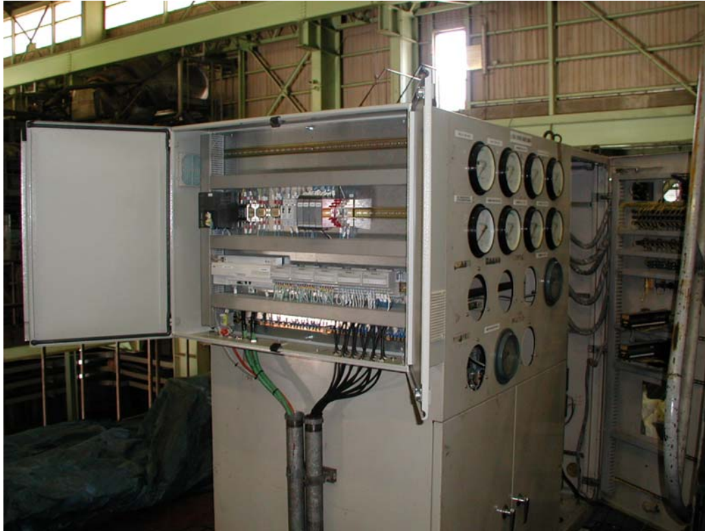
Installation of SCADA System
